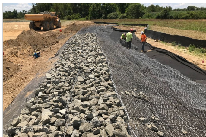
Gabion Mats being rolled out and filled
