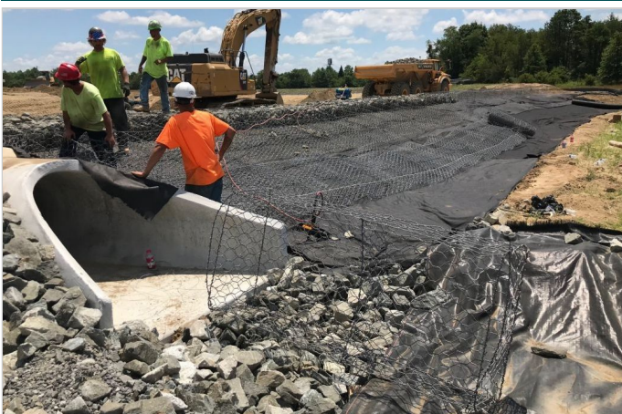
Gabion Mat being cut to fit next to concrete outlet structure
