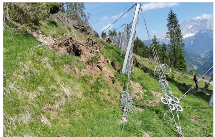
Solution details - Energy dissipating devices
