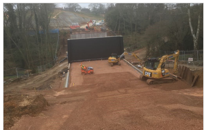
Work started on the Macwall - Jan 2018
