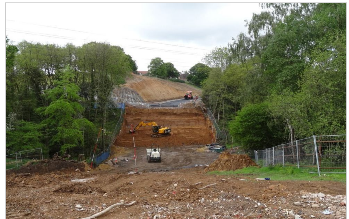
Initial earthworks towards the end of 2017
