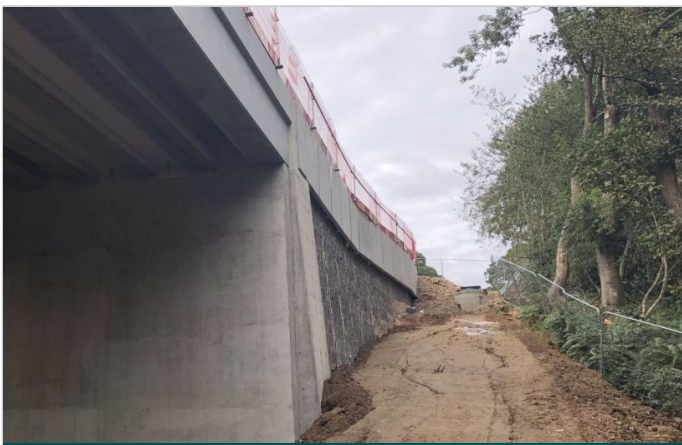
Macwall structure installed over the Paralink LTP embankment
