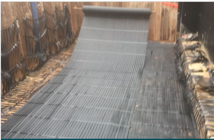
ParaLink 350 & 1100 being rolled out in a piled embankment
