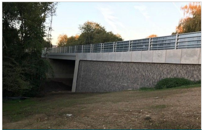
Macwall MSEW structure completed in Autumn 2018
