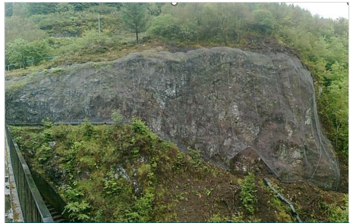
Figure 2 : Laying Down of Macmat R
