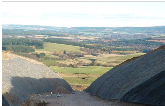
Detail looking along cutting
