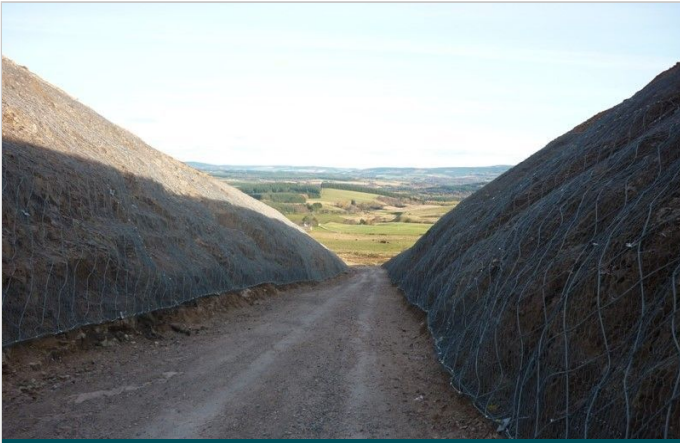
Narrow access way
