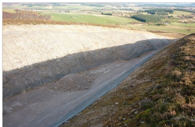
Completed Installation - HEA and DT Mesh
