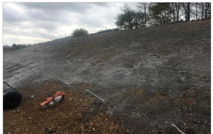
During installation of 32mm diameter soil nailing
