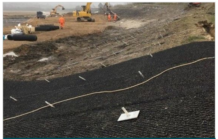
View of the site during installation
