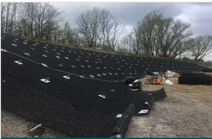
Soil nailing and MacMat® R installed
