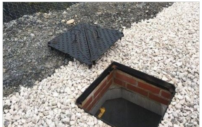
Drainage installed at the toe
