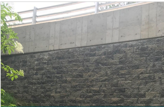
Culvert headwall below MacWall® Vertica structure
