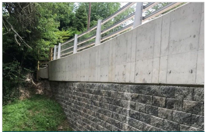
MacWall® Vertica MSE wall - side view
