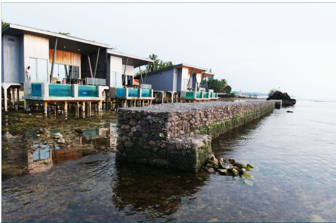
Aston Hotel Anyer Breakwater (3/3)
