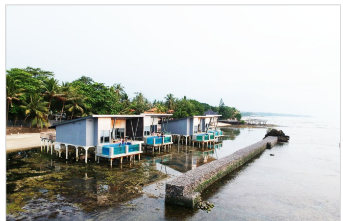
Aston Hotel Anyer Breakwater (2/3)
