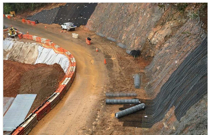
SG HR30 and erosion control mat installation in progress at upslope
