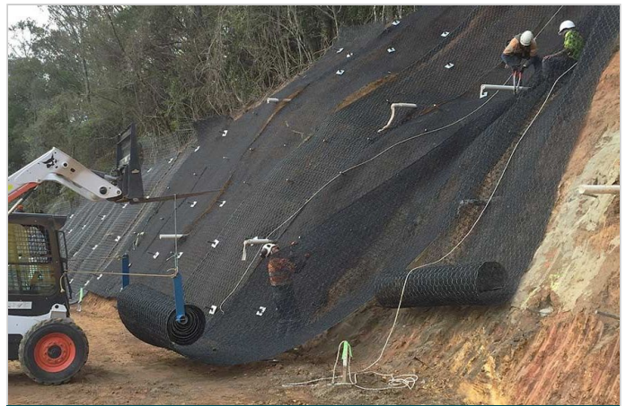
Erosion control mat installation in progress
