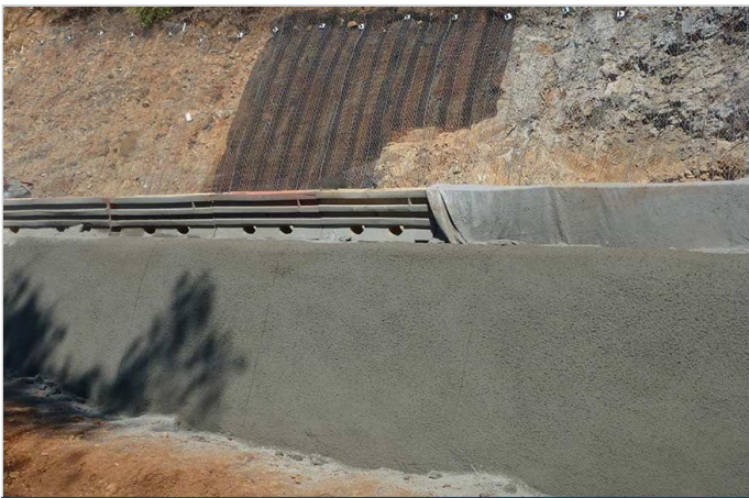
Front view of slope strengthening works upslope and downslope
