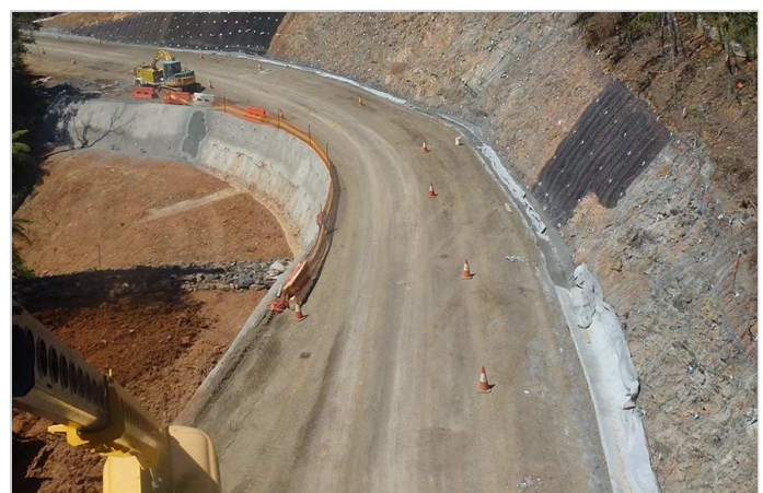
Complete installation of slope surface protection works
