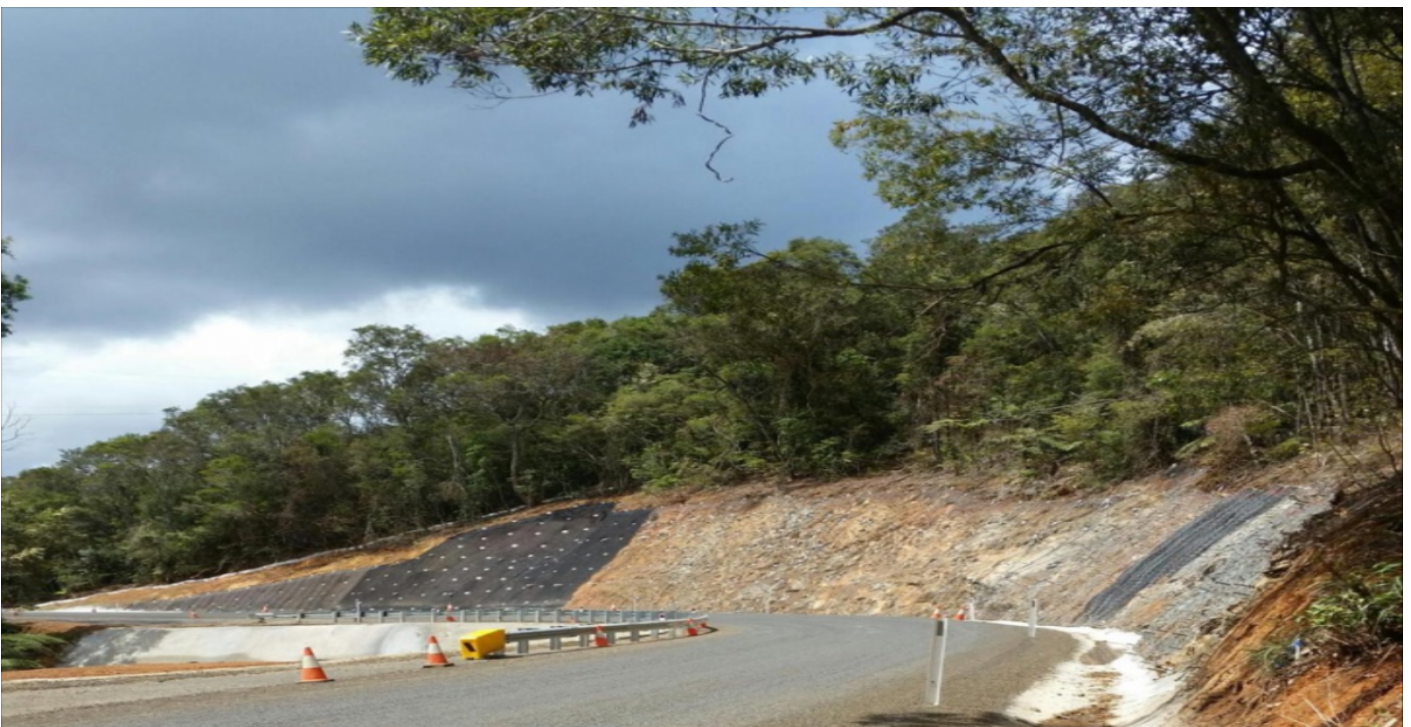
Completed rectification works
