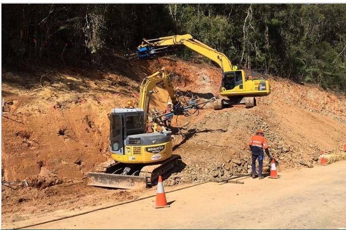
Upslope soil nail installation in progress
