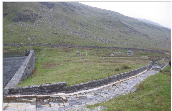
View along the dam
