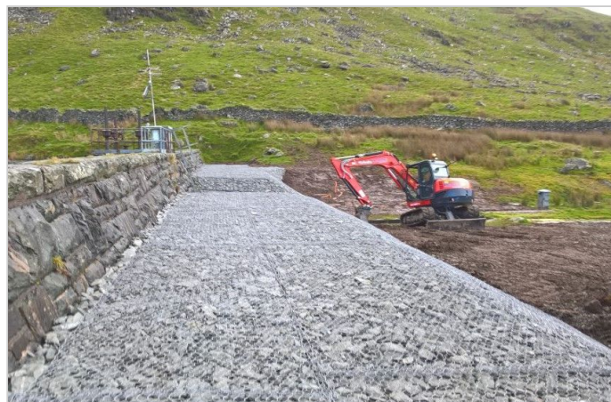
View of the Reno Mattress during construction
