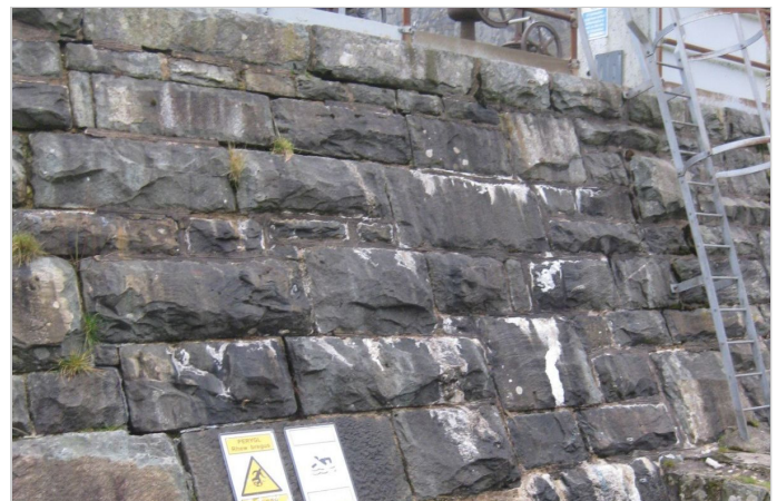
Downstream face of the dam to be supported by the proposed berm
