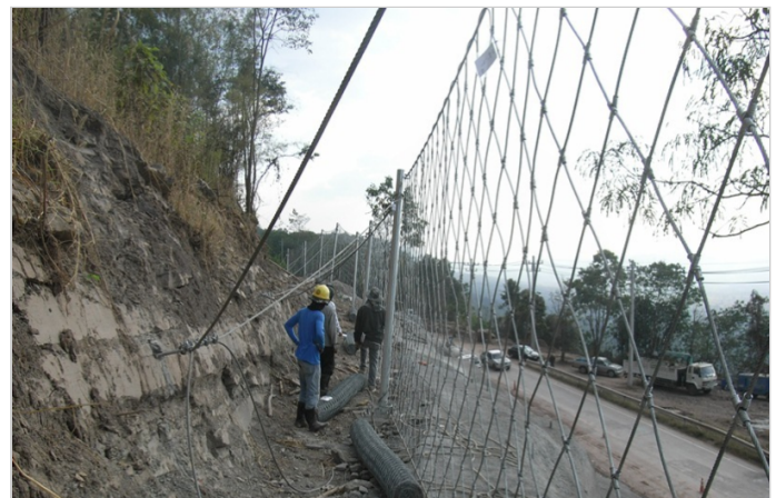
Debris Flow Barrier During Construction
