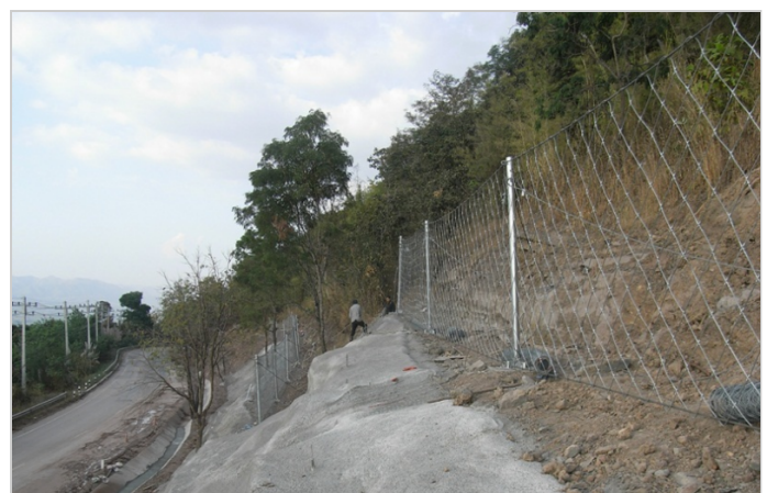
Debris Flow Barrier Construction Completed
