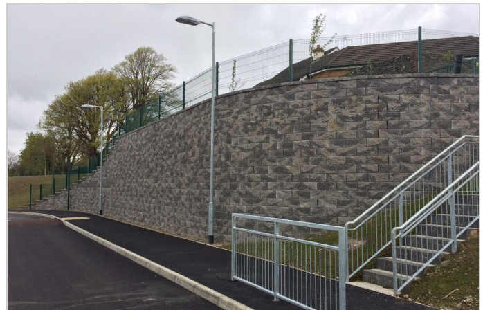
Retaining wall near stairway to the school
