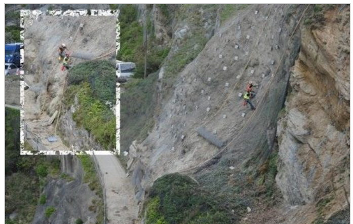
Abcas was installing the Maccaferri solution
