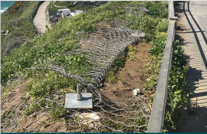
Steelgrid HR secured at the crest of the cliff
