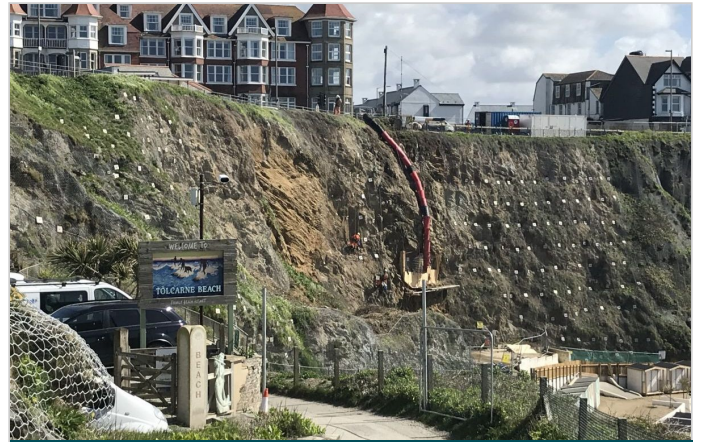
View of the works in Autumn 2017
