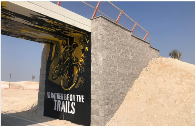
Completed MacWall (Bridge no. 4)
