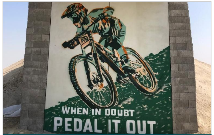
Completed MacWall (Bridge no. 3)
