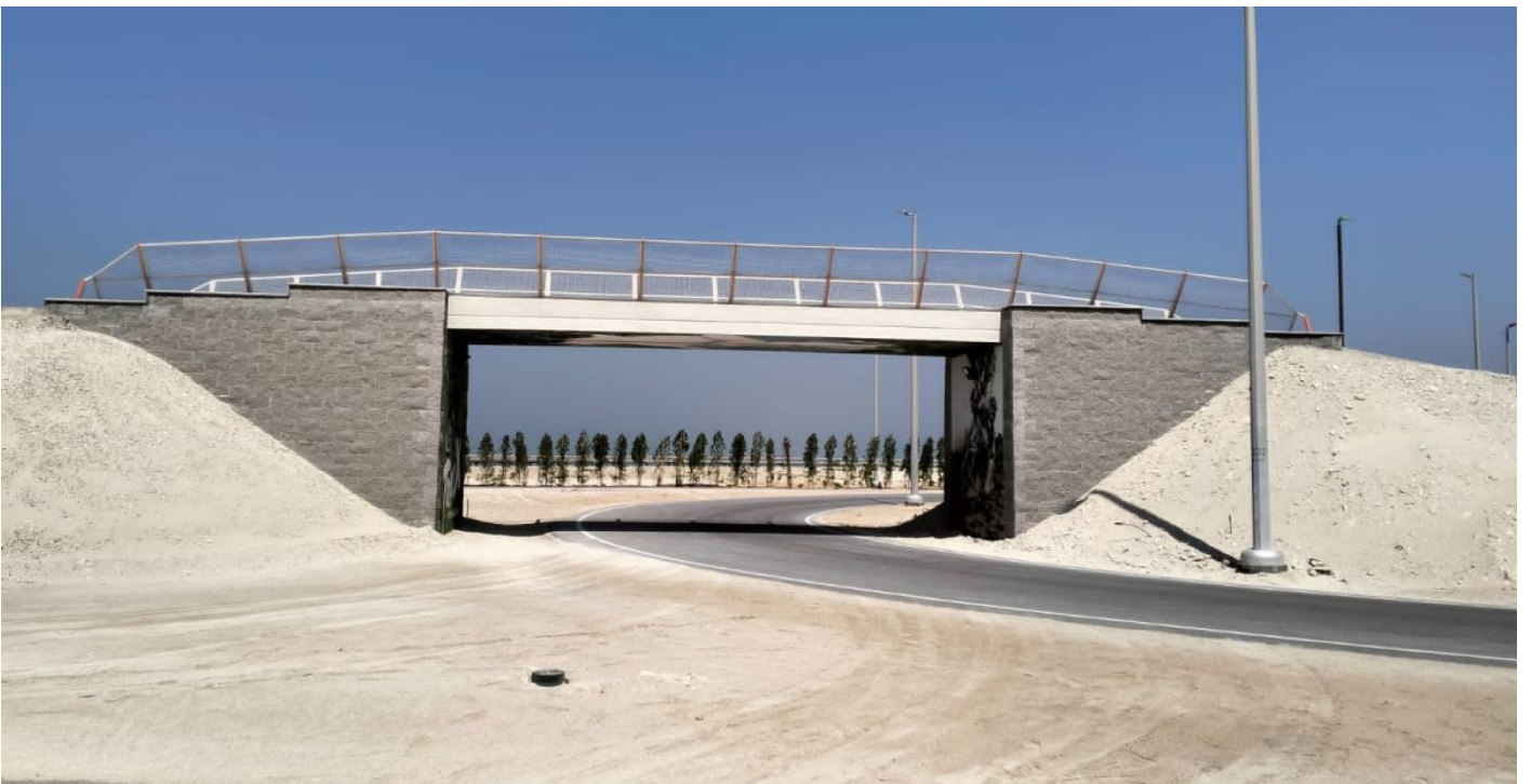
Completed MacWall (Bridge no. 6)
