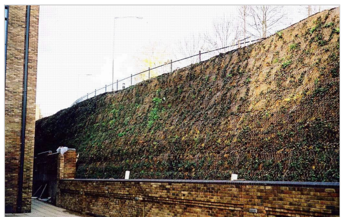
Soon after construction Date: November 2001
