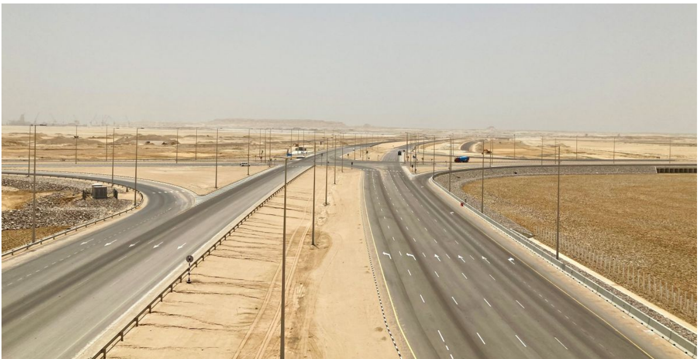
Completed roads stabilized with ParaLink high strength geogrids
