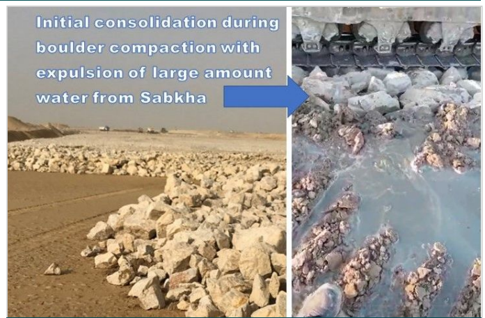
Various stages of boulder laying
