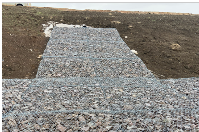
Reno mattresses installed at pond outfall.
