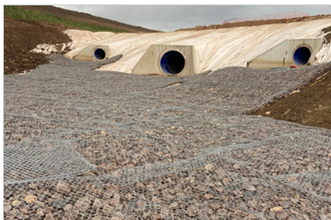
Mesh can be locally cut and shaped
