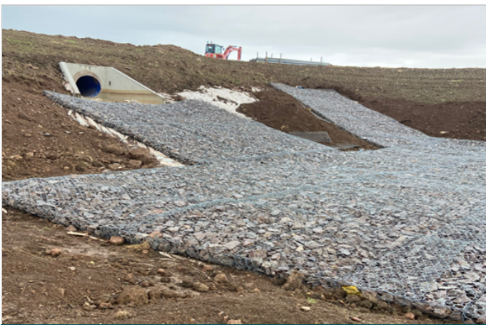
Reno mattresses can be installed on slopes up to 45 degrees
