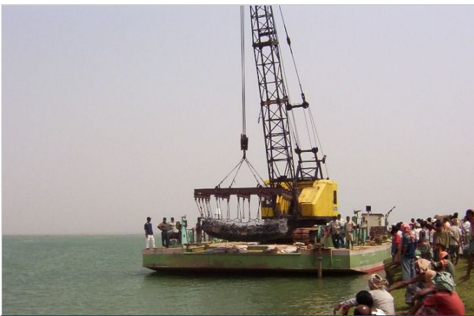
Photo 3: Pre-filled mattress lifted and taken in the barge
