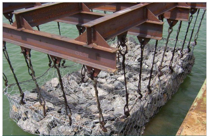
Photo 4: Lowering the units for under water placement
