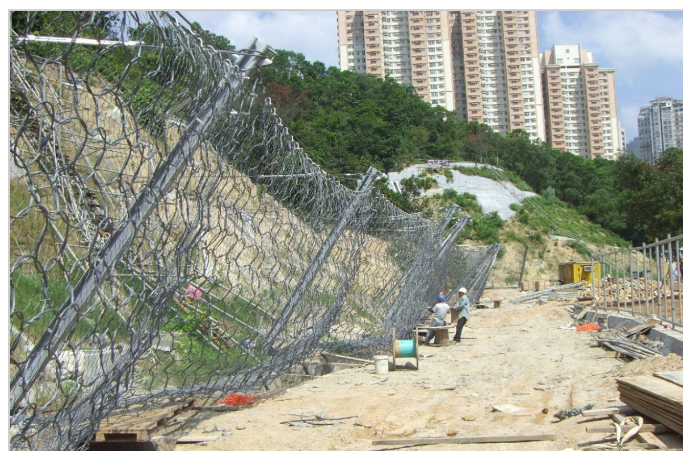
Installation of dynamic barrier in progress (view from downslope)
