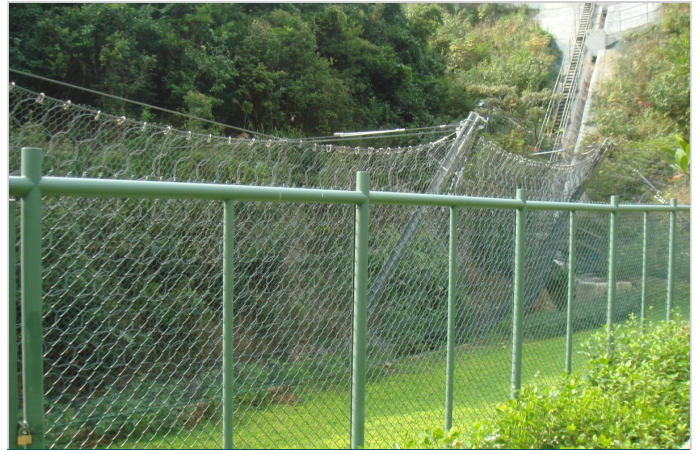
Complete installation of dynamic barrier (view from downslope)
