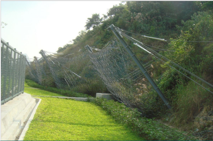
Complete installation of dynamic barrier (view from downslope)
