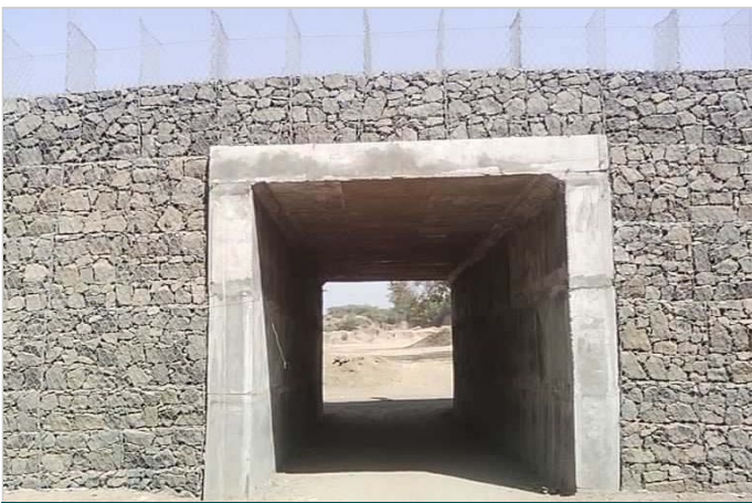
Photo 3: Construction stage- Terramesh system with box culvert
