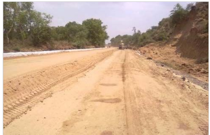
Photo 1: Initial stage of construction
