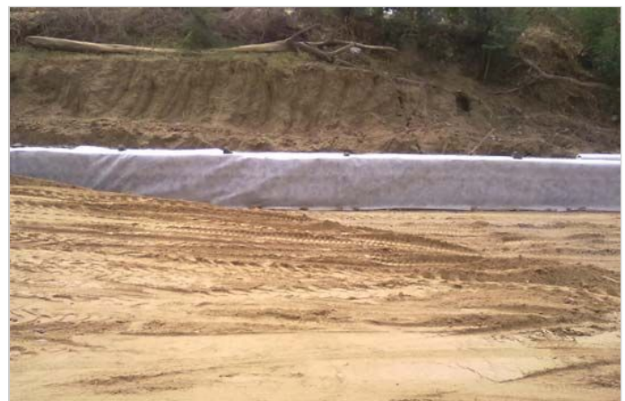
Photo 2: Terramesh system wrapped with geotextile
