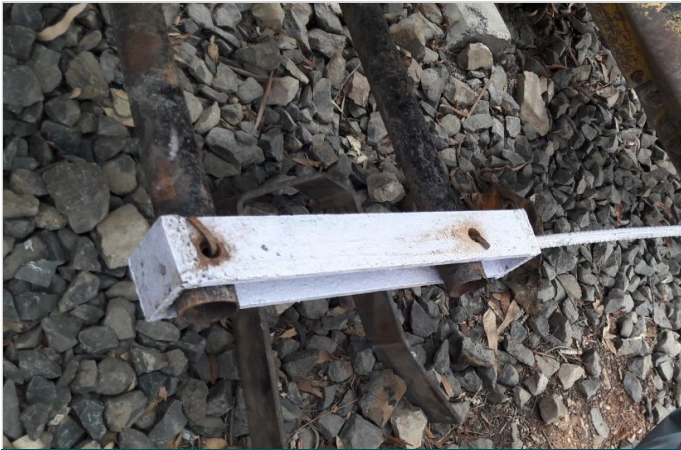
Photo 3 : Fixing of rode for unrolling the MacGrid & MaxTex
