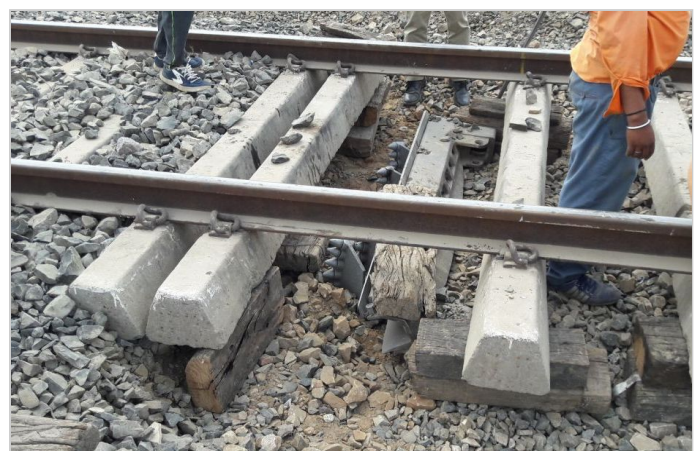
Photo 2: Lifted Sleeper supported using wooden planks
