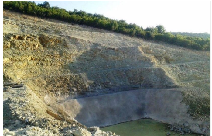
Istanbul - Şile - Agva Road V4 Viaduct Slopes
