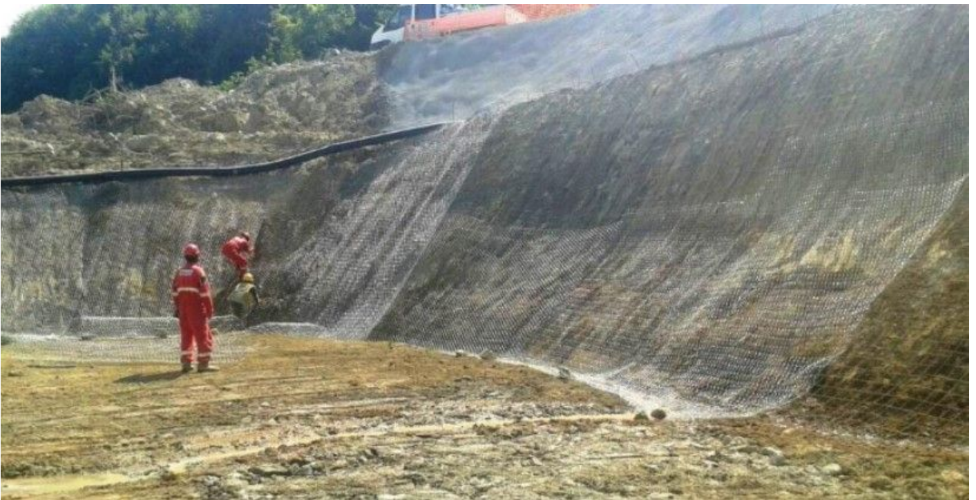
V4 Viaduct Rockfall Protection Measures
