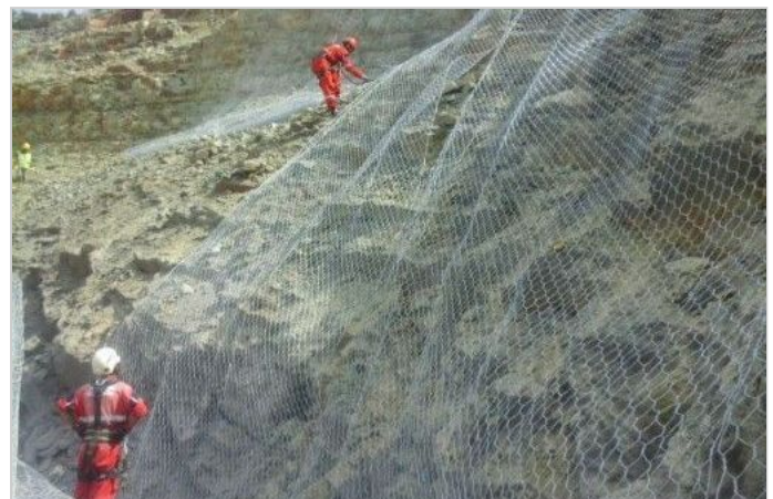
V4 Viaduct Rockfall Protection Measures
