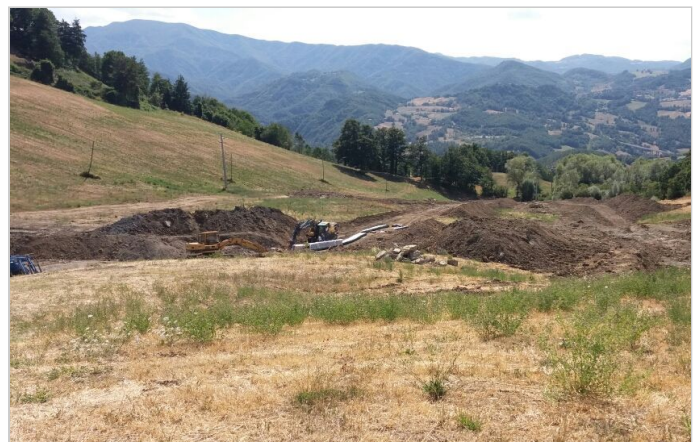
Posa in opera trincea drenante
