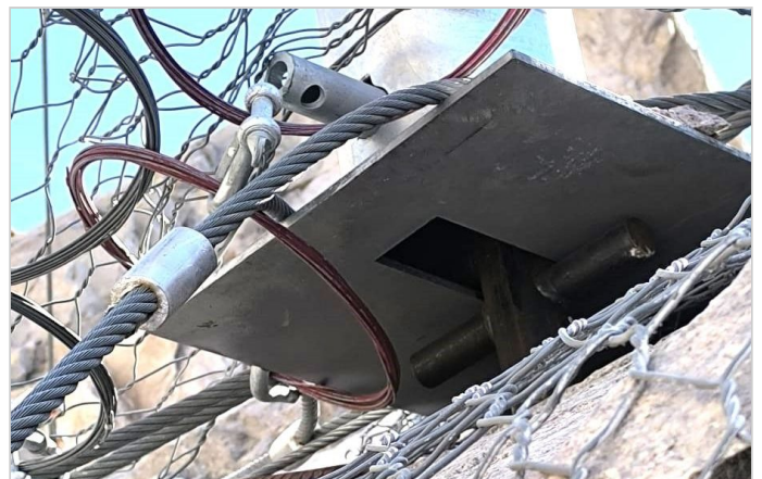
Base plate kept in level using micro-pile
