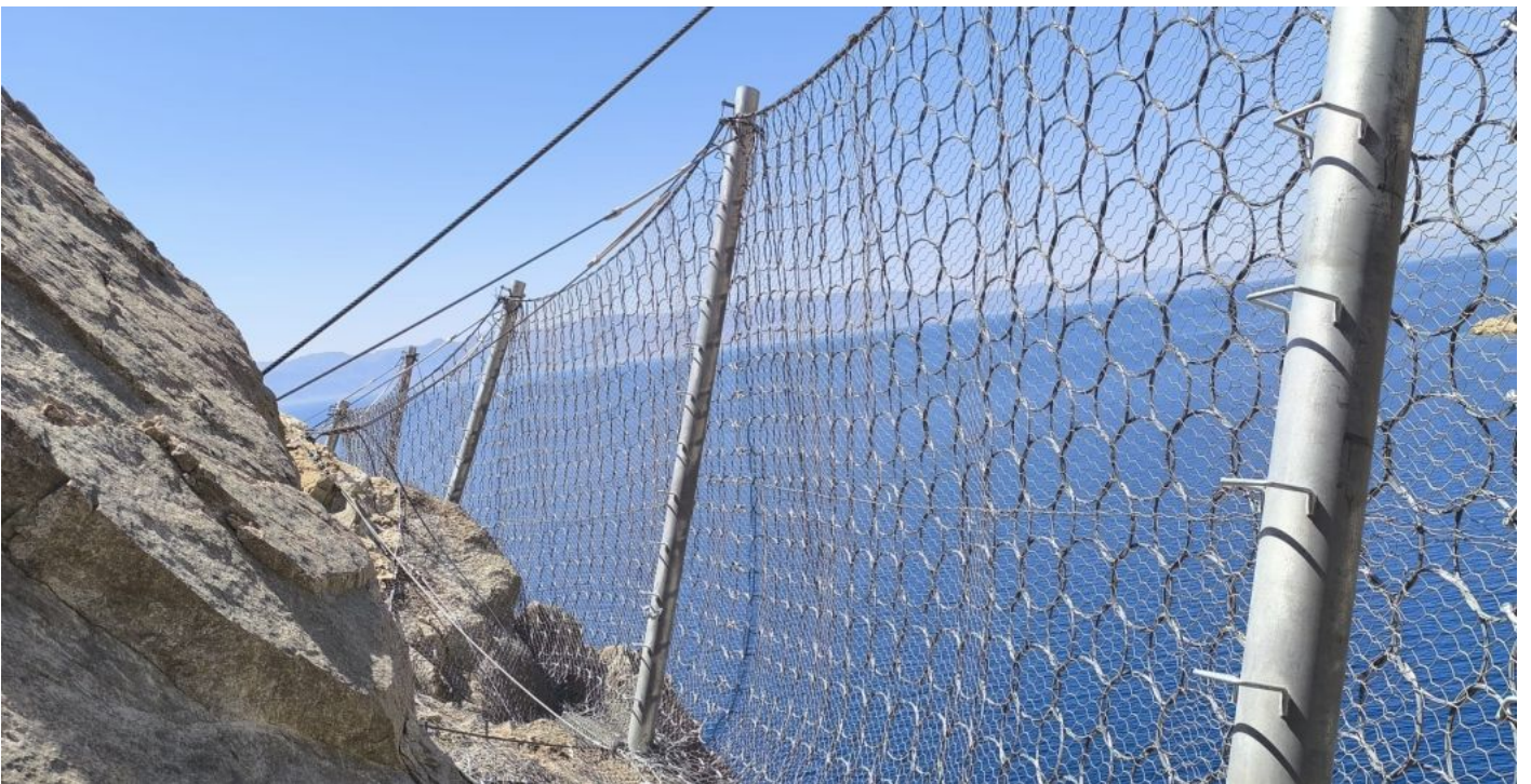
Completed rockfall protection barrier in one of the locations of the project
