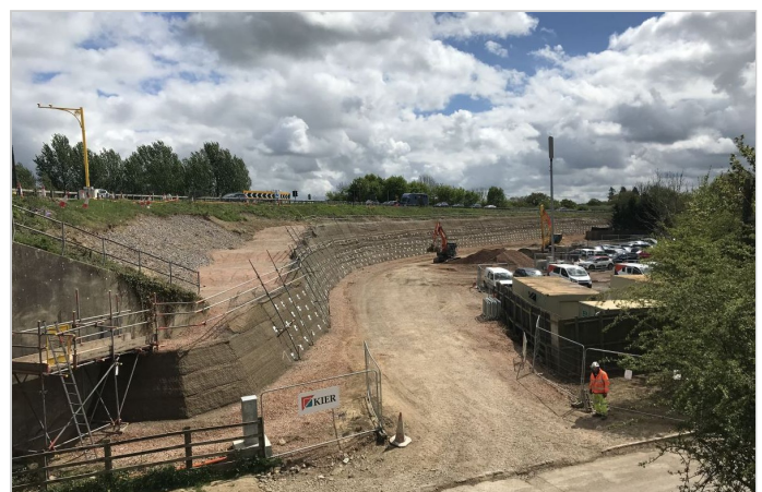
Green Terramesh with soil nails installed
