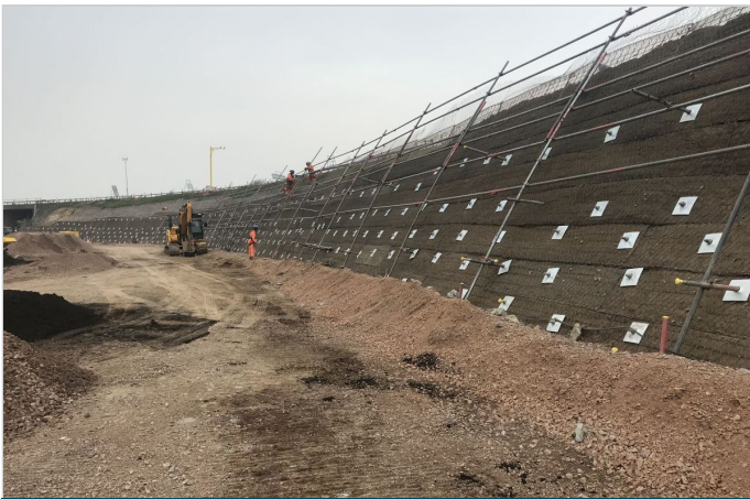
Green Terramesh and soil nails during construction
