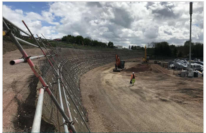
Green Terramesh and soil nails during construction
