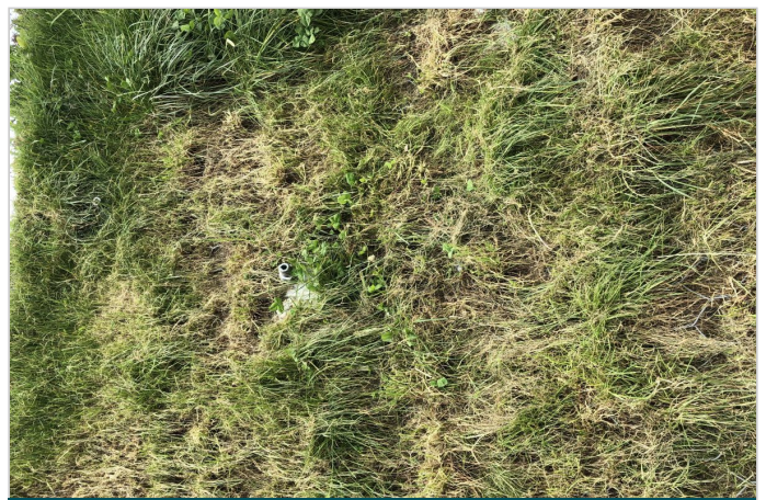
Vegetation established in Green Terramesh - note nail head
