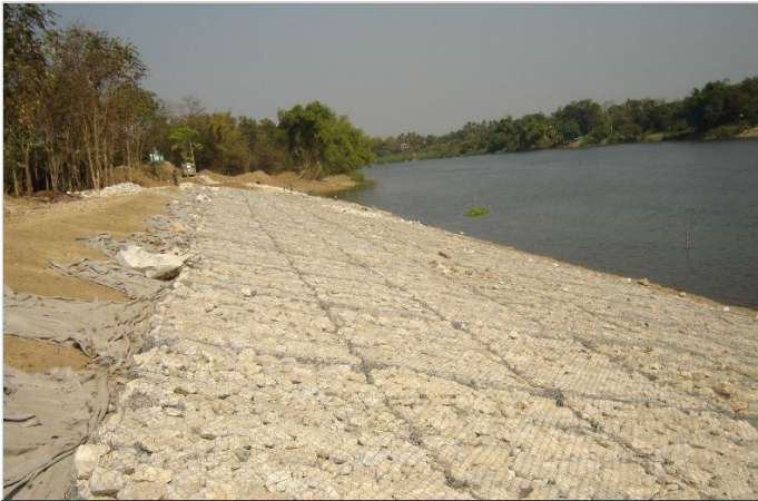
Reno Mattresses revetment (3)
