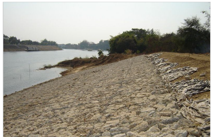
Reno Mattresses revetment (1)
