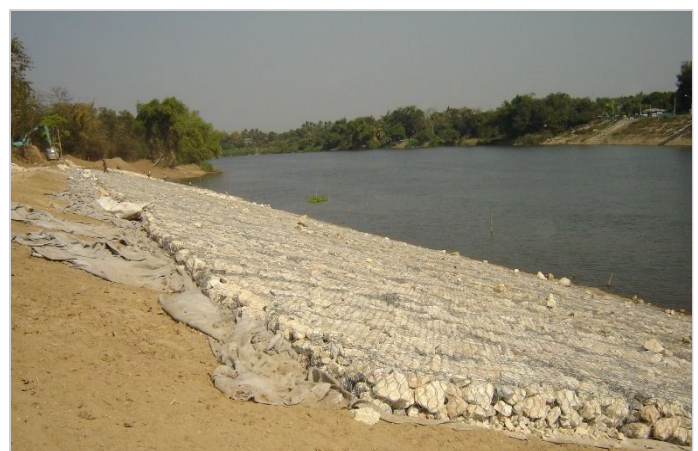
Reno Mattresses revetment (2)
