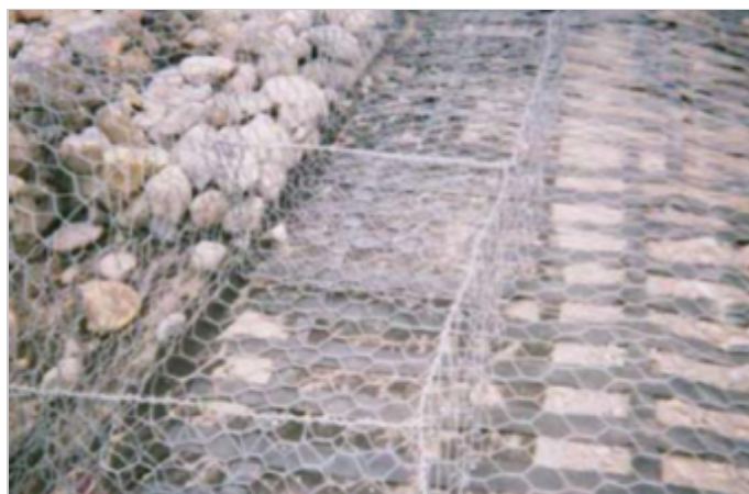
Detail of Paralink® sandwiched beneath Terramesh® unit (unfilled)
