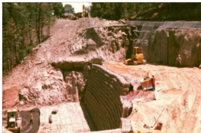
Compacting structural backfill onto the Paralink® and Terramesh®
