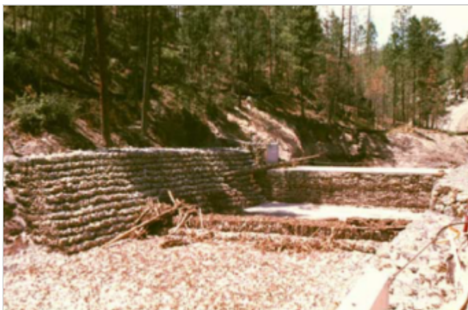
Gabion and Gabion mat® revetment, and debris basin
