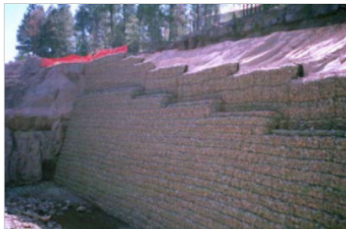
36' high MSE structure supporting North Road
