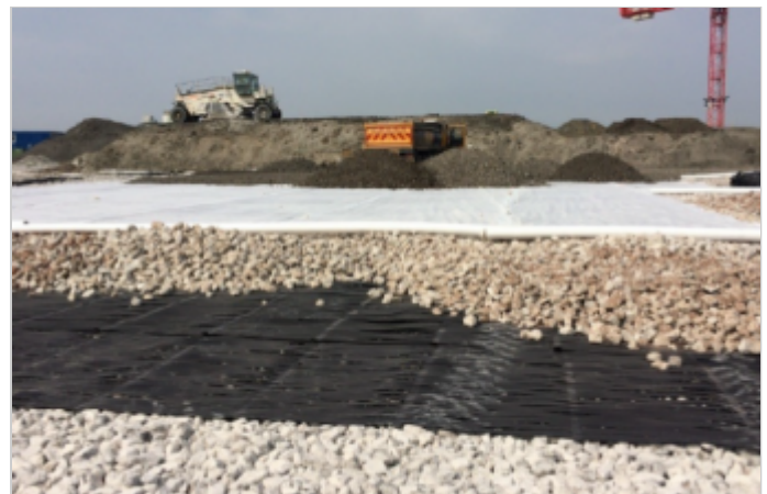
Paralink underneath the embankment over soft soil
