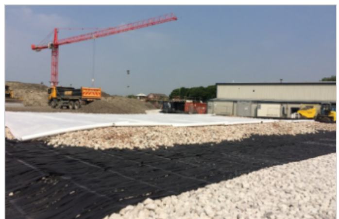
Paralink underneath the embankment over soft soil
