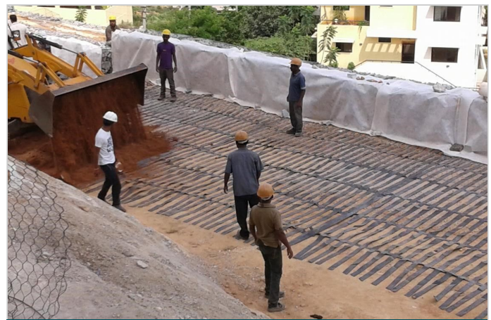
Figure-4 Top wall-During construction-Laying of Paralink
