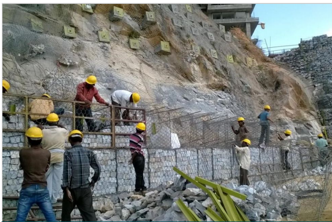
Figure-3 Top wall-During construction-Gabion installation
