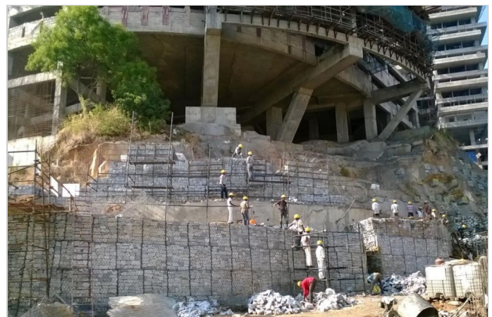
Figure-2 Top wall-During construction-Gabion installation
