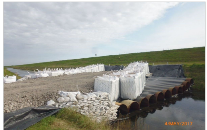
Initial phases of the works
