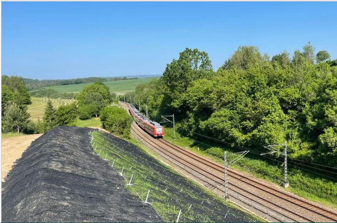
Railway still working during the installation phase
