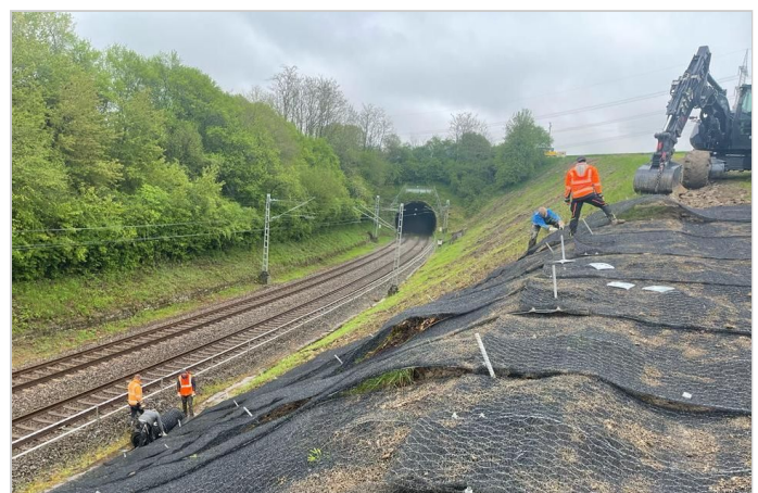
During the installation
