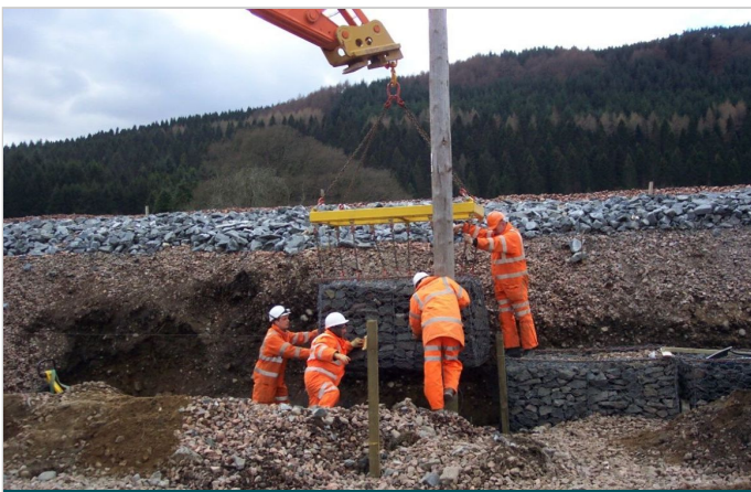
Installation in progress
