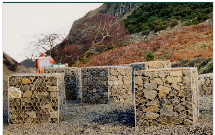
Pre-Filled Gabions in the quarry
