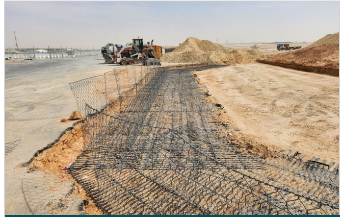
Laying of first layer of Terramesh facia unit
