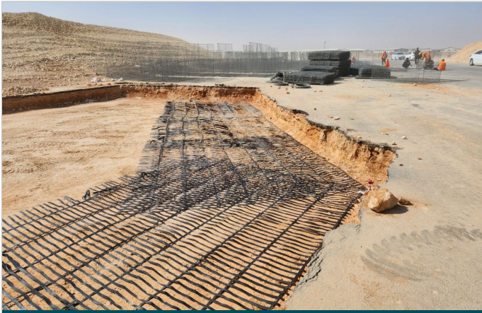
Laying of first layer of Paragrid geogrid
