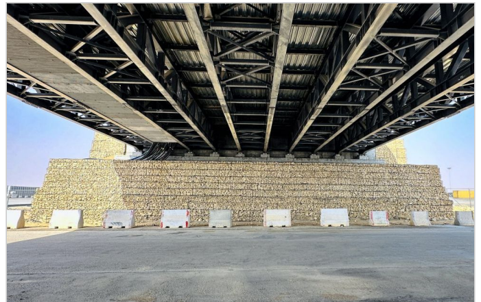
Completed: View of Paramesh wall below the bridge
