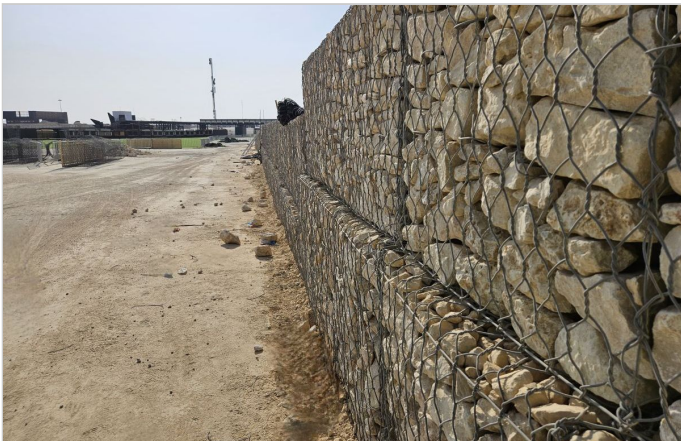
Paramesh wall in progress
