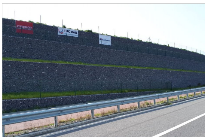
After the construction: side view detail
