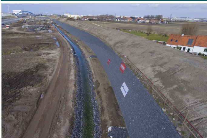
Construction phase: drone view
