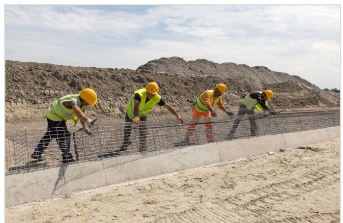
Detail of the welded gabion wall
