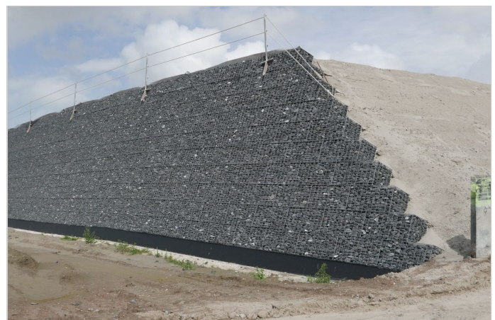
Construction phase: side view detail
