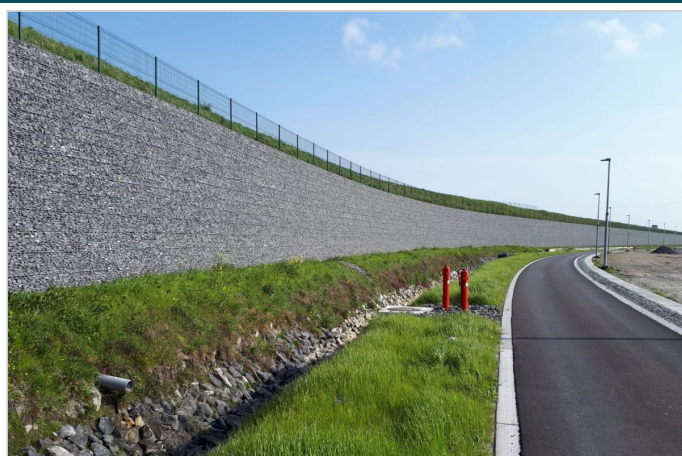
After the construction
