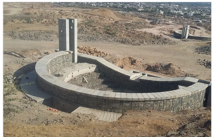
Photo 1: Series of check dams under construction
