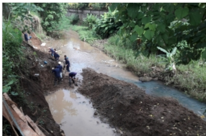
Start of Construction
