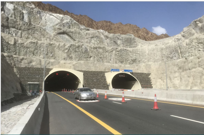
Completed Terramesh wall at Al Saha Tunnel
