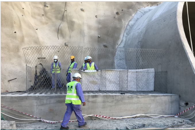
During construction: Initial layer of Terramesh and Paralink geogrid placed
