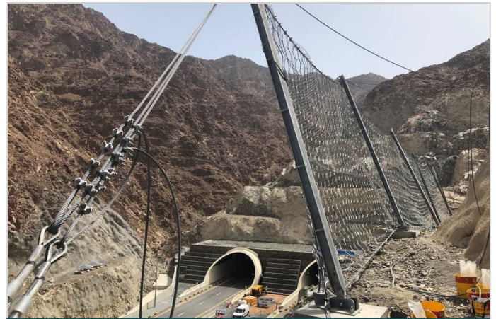
Maccaferri Rockfall Barrier installed at one of the tunnel locations
