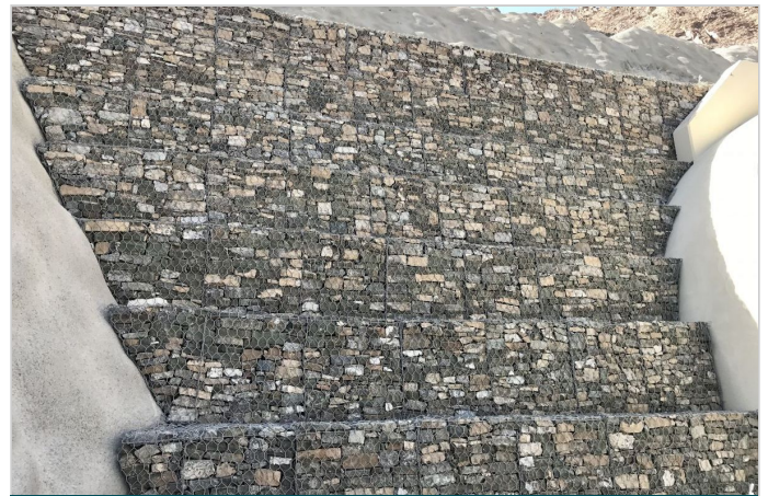
Close view of completed Terramesh wall at 1 location (out of total 10 locations)
