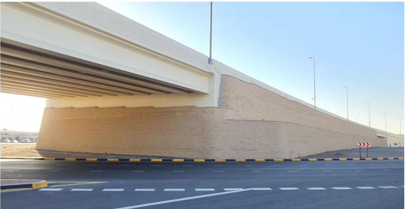
Completed MacWall MSE wall at Al Madam Roundabout
