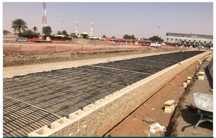
Paragrid geogrid connected to fascia blocks
