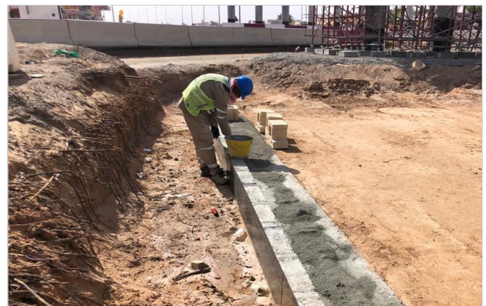
Concrete levelling pad laying
