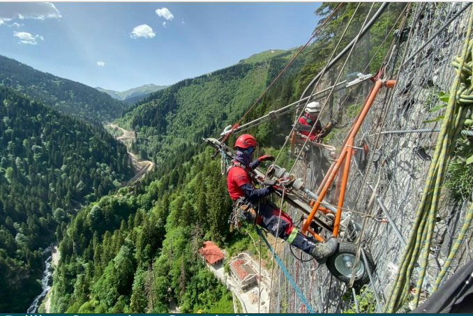
Drilling Operations Sumela Monastery
