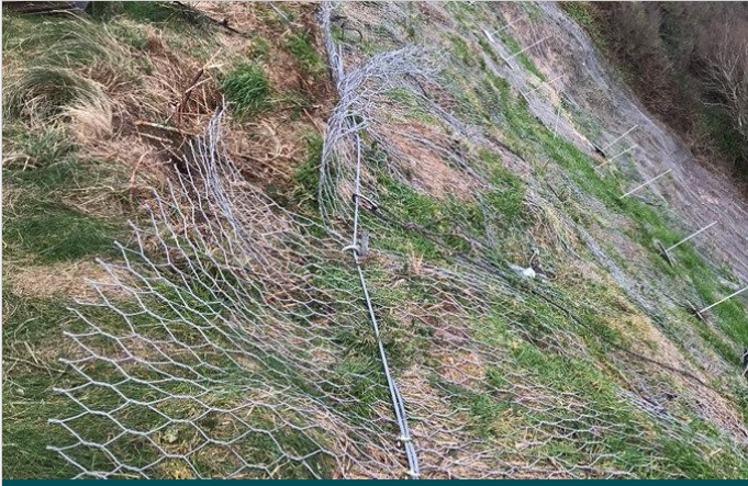
Installation of anchors and crest rope secure the DT netting
