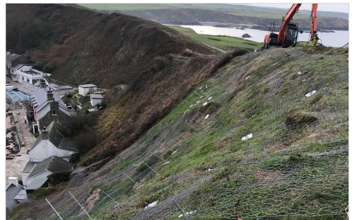
DT Rockfall netting being secured to the cliff slope.
