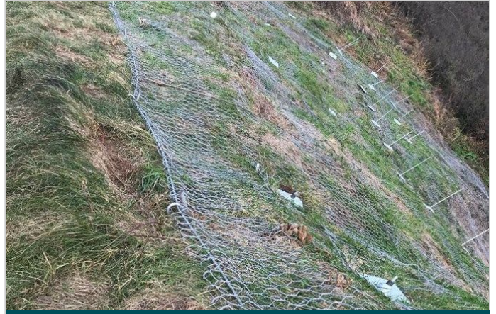
The DT netting is wrapped back over the crest rope & secured
