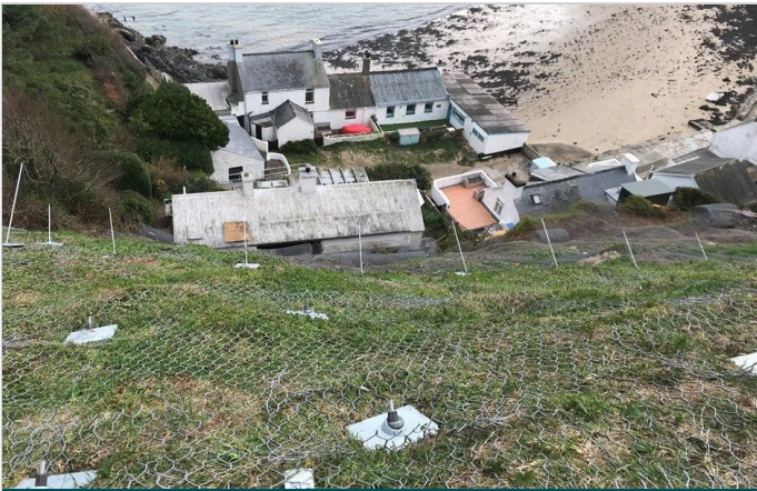
Polimac DT rockfall netting successfully installed
