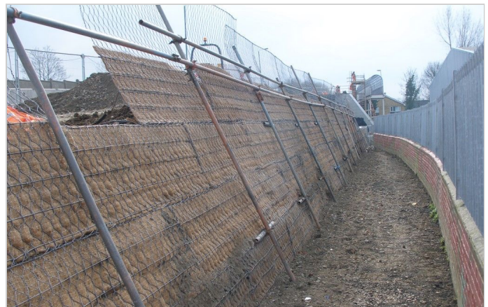
Green Terramesh® after installation
