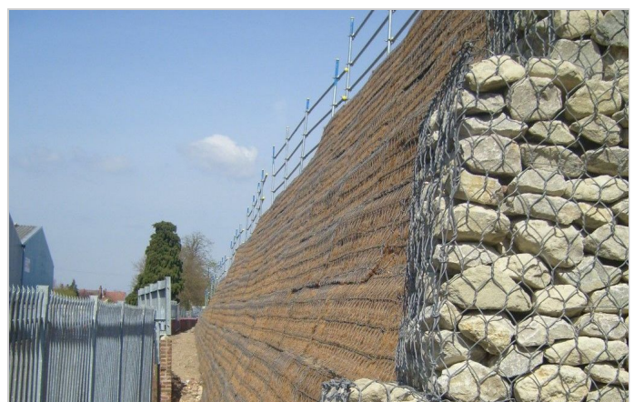
Green Terramesh® with Gabion Terramesh Wall
