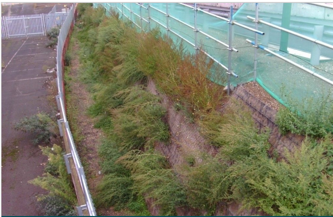
Two months after installation
