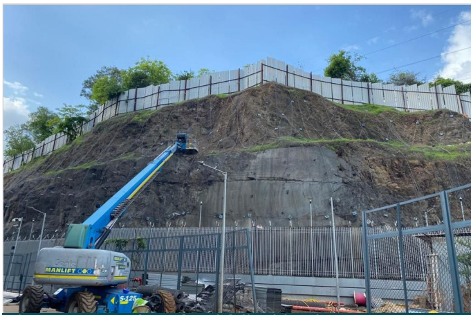
Figure 5 Execution of rockfall mitigation measures
