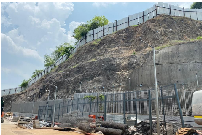
Figure 2 Execution of rockfall mitigation measures
