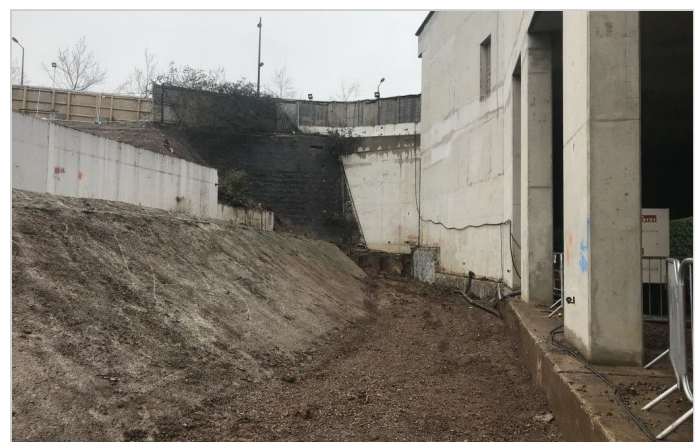
Formation of the working platform
