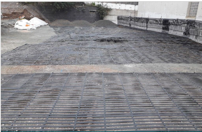
Paragrid laid in layers to form the Parawall System
