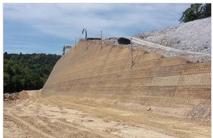
Muro in Terramesh Verde
