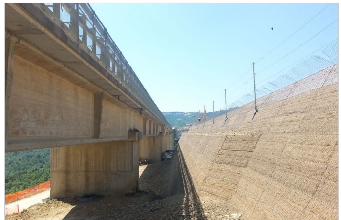
Muro in Terramesh Verde
