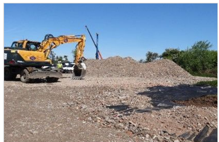
Granular material placed upon MacTex W1
