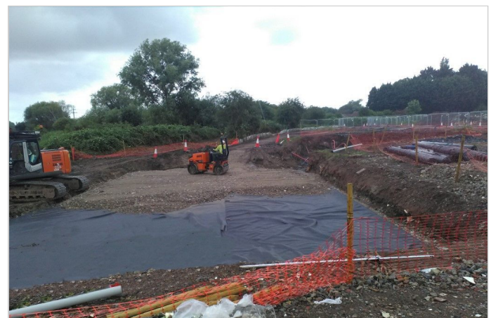
MacTex W1 S laid over soft clay sub-strata
