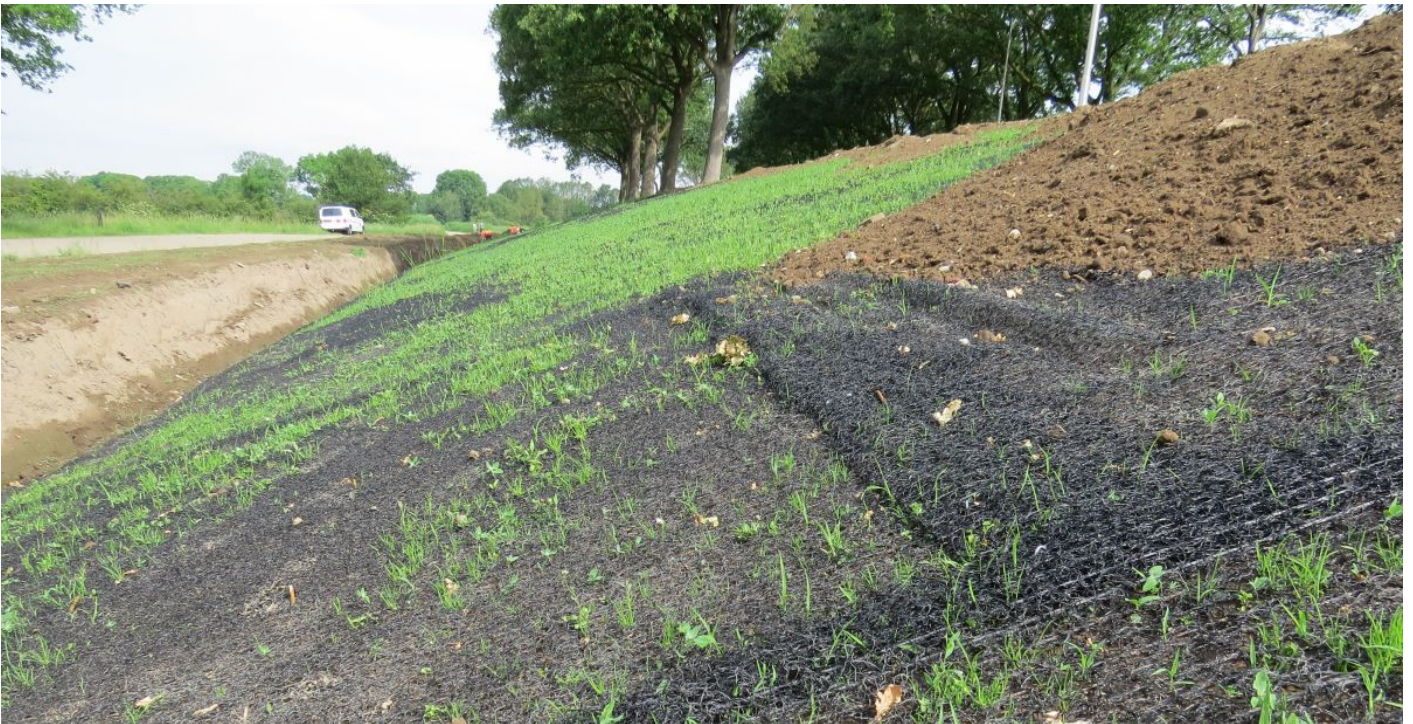
Detail of the MacMat before the laying of the vegetative soil
