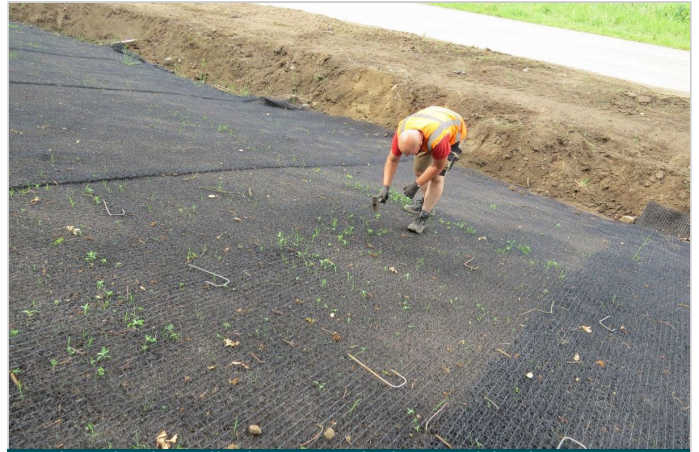
During the installation: metal pins positioning
