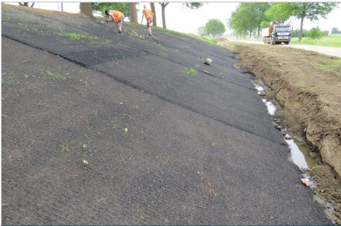
End of installation
