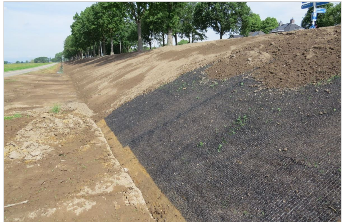
After installation: vegetative soil layer
