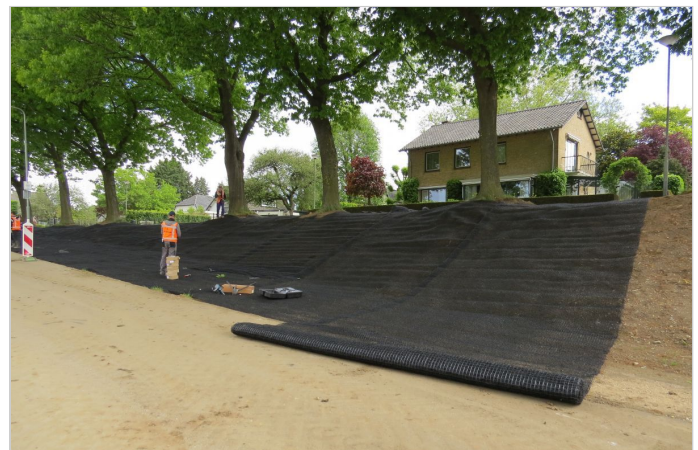
During the installation: unrolling phase
