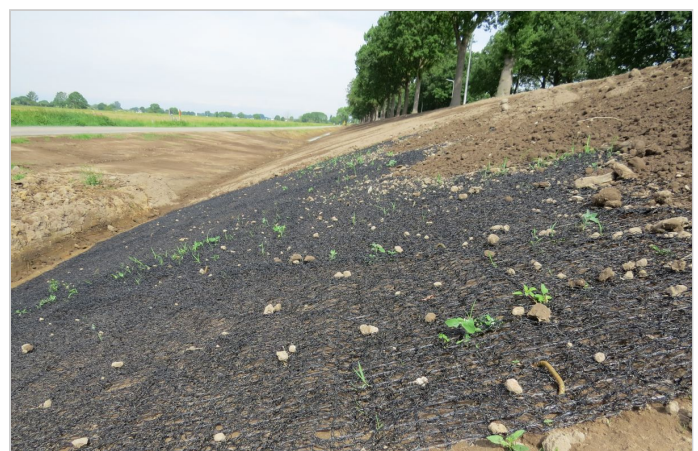
During the installation: side view
