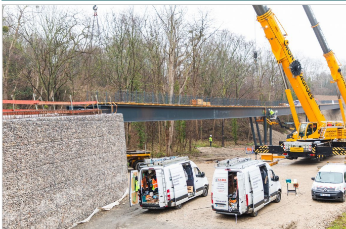
Rampe Passerelle Terramesh System
