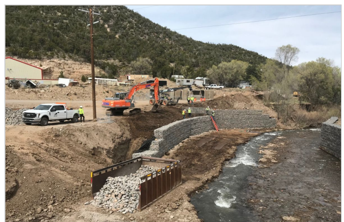
Gabion Installation
