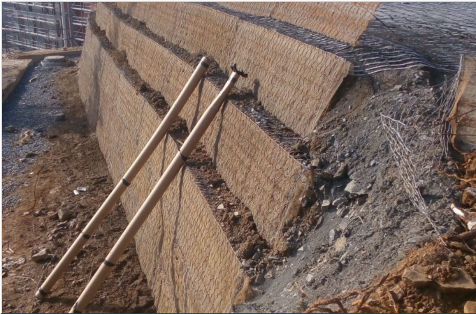
Torunkent 5.Levent Project GTML Application
