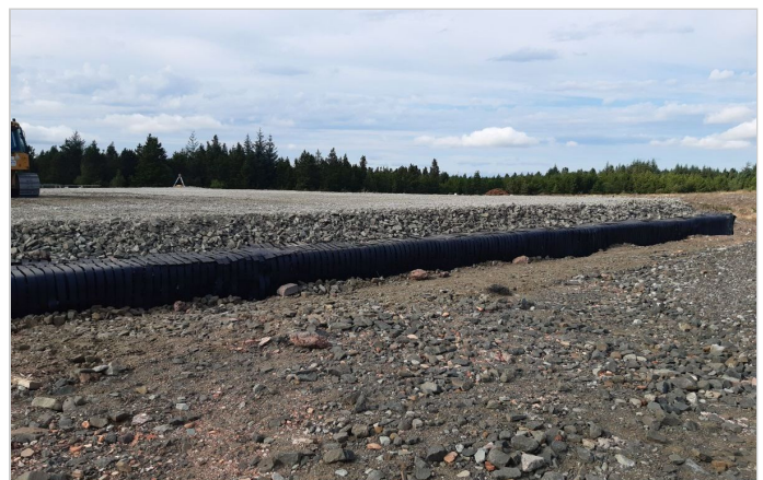
ParaLink Installation for work platform
